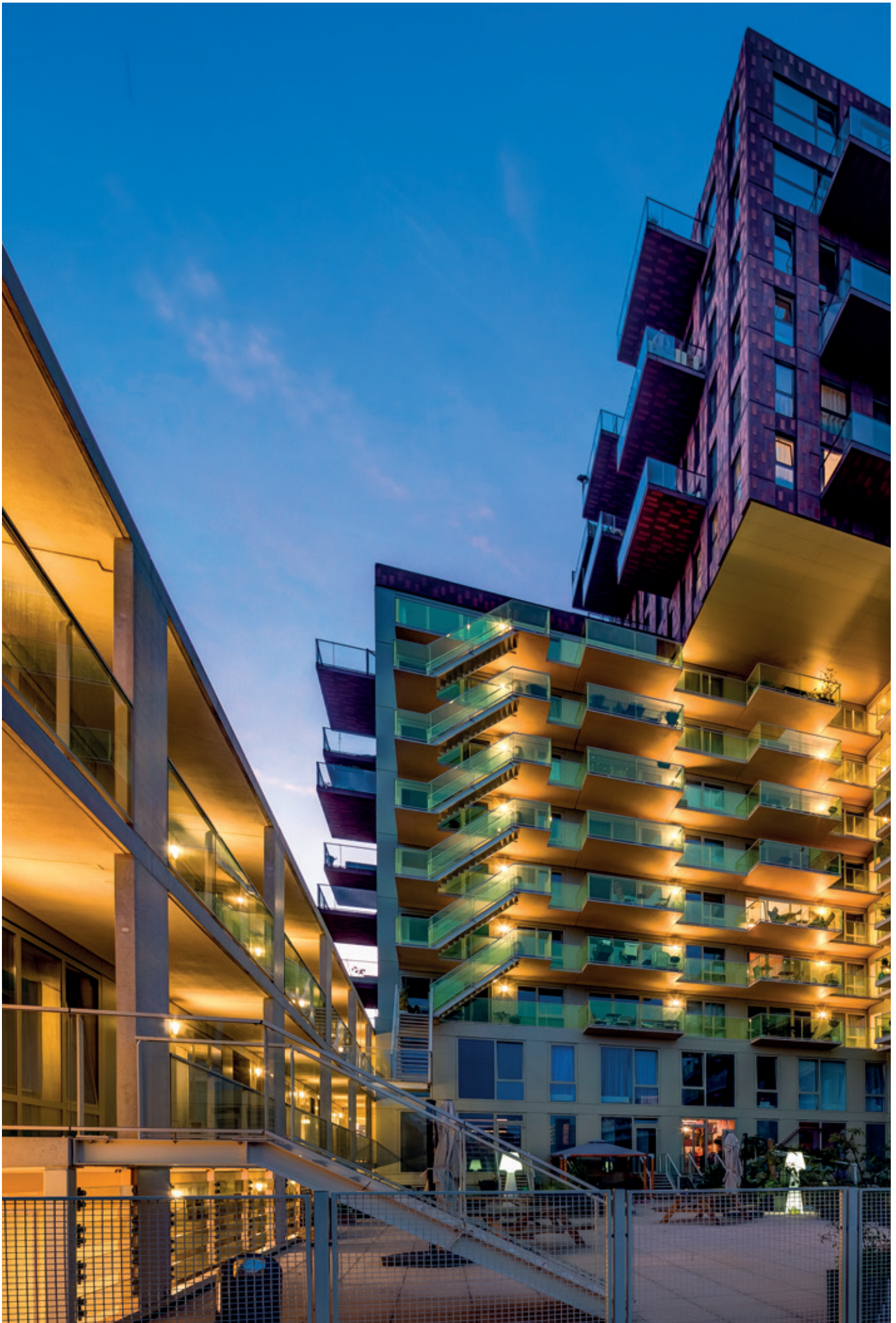
Residential Tower De Verkenner - Utrecht - Netherlands
