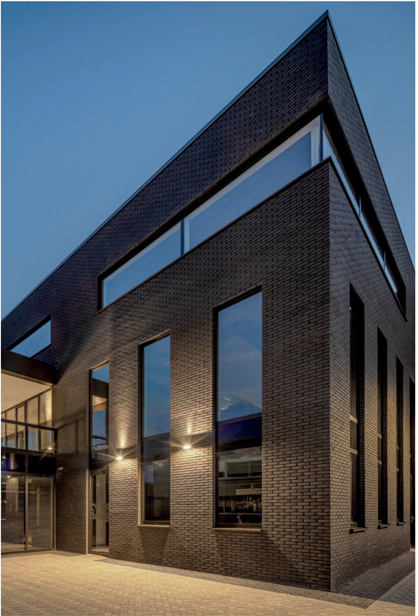
New Building Electrical Wholesaler Robri - Wekerom - Netherlands
