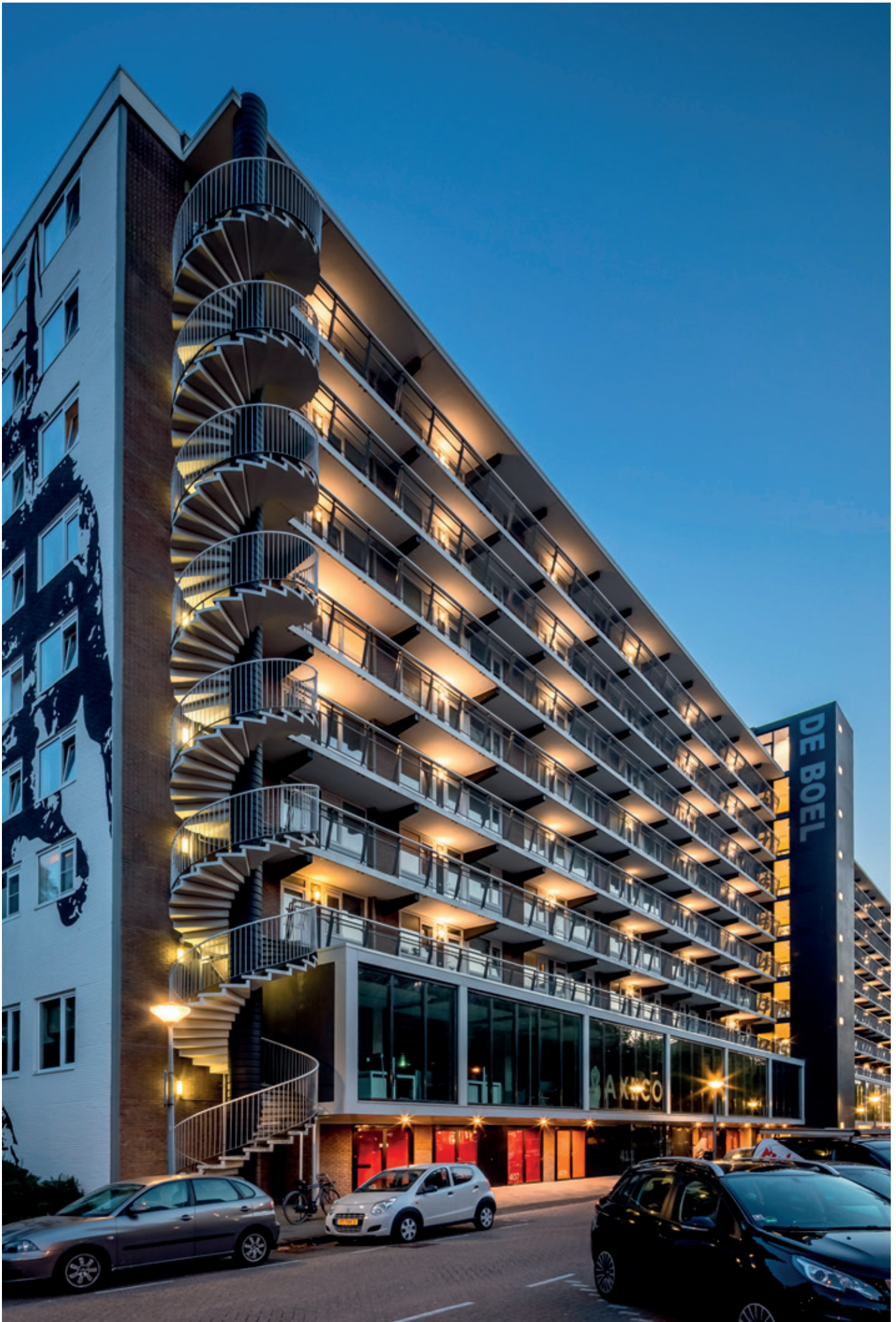
Apartment building De Boel - Amsterdam - Netherlands
