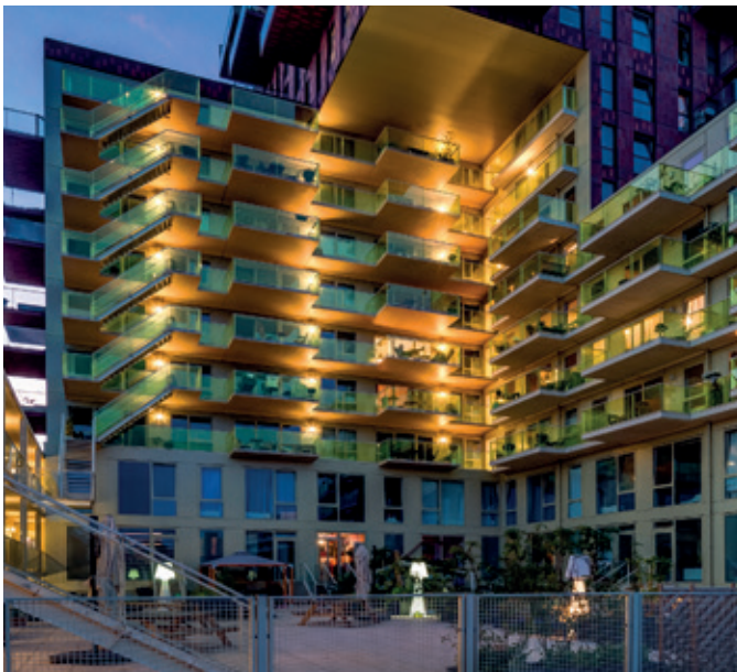
Residential Tower De Verkenner - Utrecht - Netherlands
