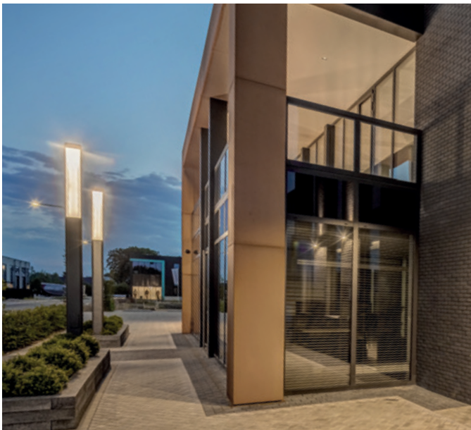
Robri - Wekerom - Netherlands
